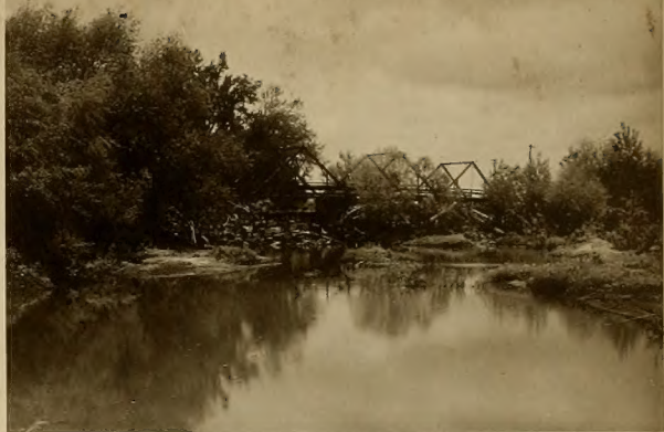
Bridge and Dam.
